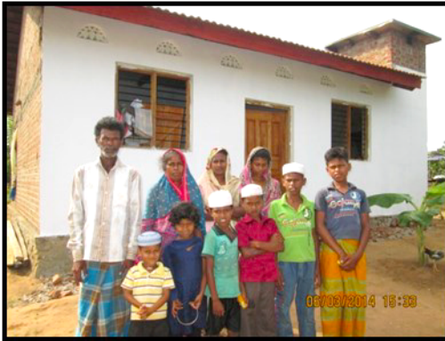
Kalantharumma's nearly complete new home
