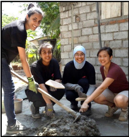
Mixing cement to plaster the walls of a house
