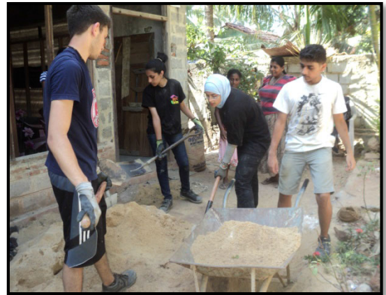
Transporting sand to make concrete
